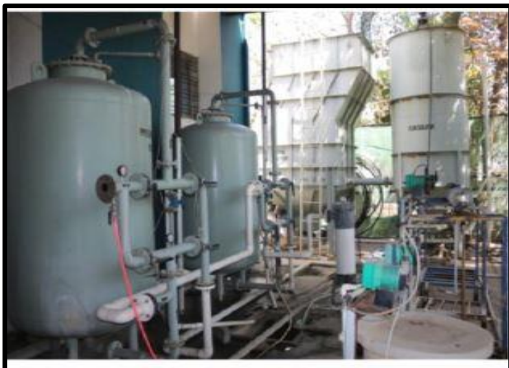
Water filter and RO Purification plant
